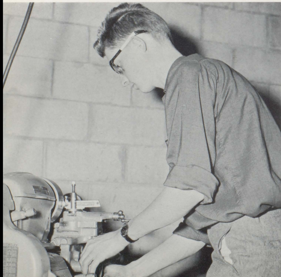
Making a screw driver handle on an engine lathe, David Hargis, one of the boys in vocational machine shop, finds this class very practical for a future career.
