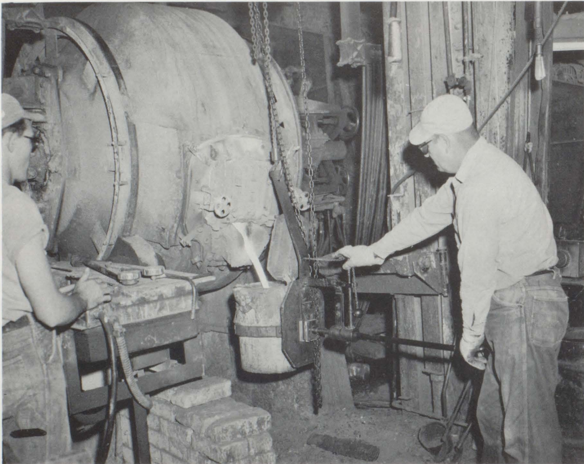
Two Perfect Circle employees are pouring molten iron from an electric furnace into a ladle. The iron is then poured into sand molds for castings.
